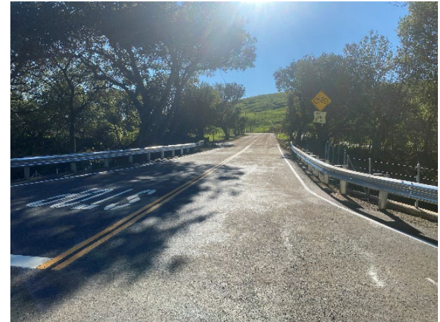
Buhman Ave. Bridge Replacement →
