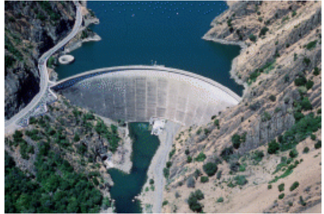
Monticello Dam – Napa County, CA
