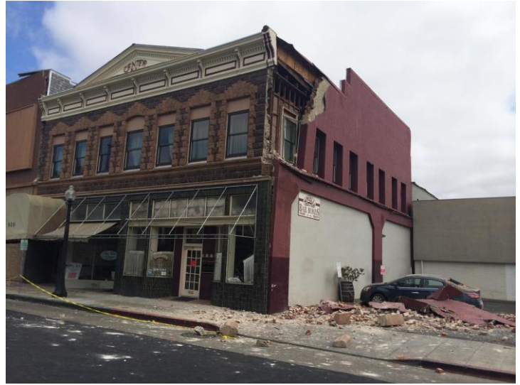
2014 South Napa Earthquake damaged unreinforced masonry building on Main St. in Napa Downtown. Courtesy of USGS
