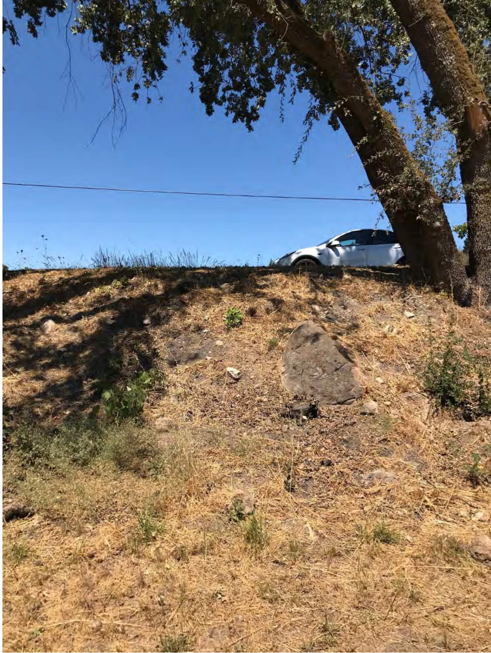
Photo #8: View of grade differential between the parcel south of the Duckhorn driveway and Lodi Lane looking north toward the Duckhorn driveway. Note grade differential and proximity of trees to roadway. This area is within the Napa River floodplain/floodway.
