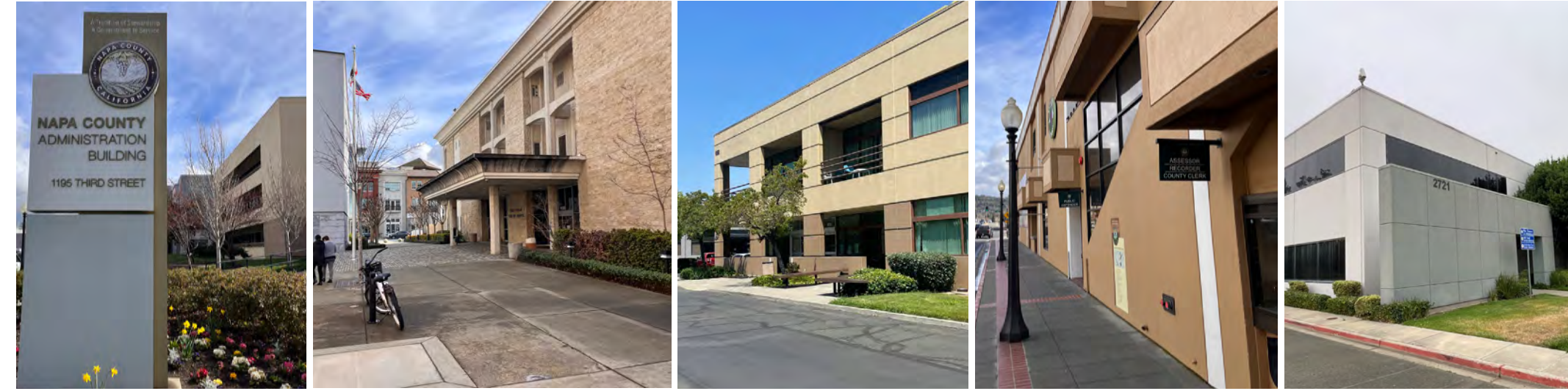
From left, County Administration Building, Hall of Justice, 650 Imperial Way, 1127 First Street, South Campus Building 4
