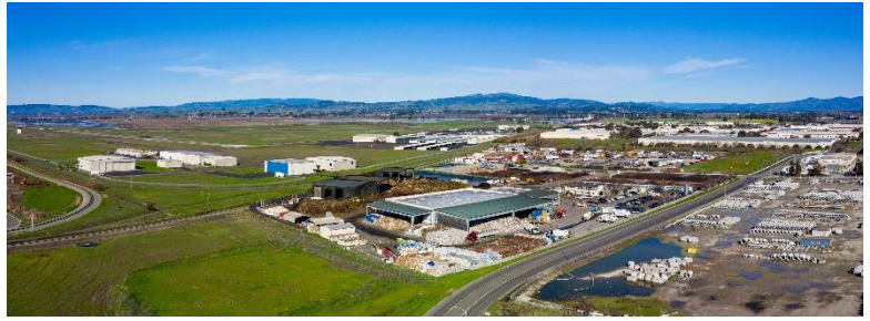
Napa Recycling and Waste Services Facilities. Courtesy of the Napa Recycling and Waste Services Website
