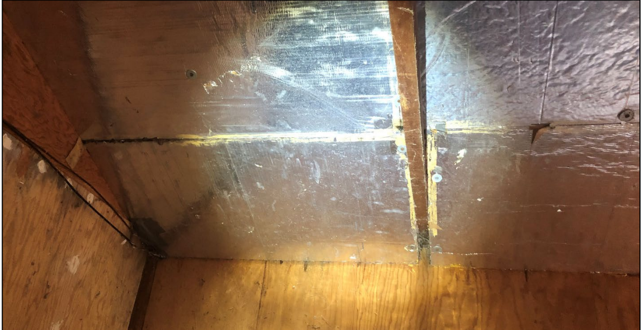
Photo 1: Looking at a typical section of roof inside the workshop. Insulation is held tight against the roof, eliminating interstitial spaces that might be occupied by bats. The workshop is also open with barn doors on either end that let in ample light and the area is regularly disturbed by workers.
