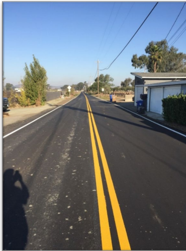
← Milton Road (Paving)
