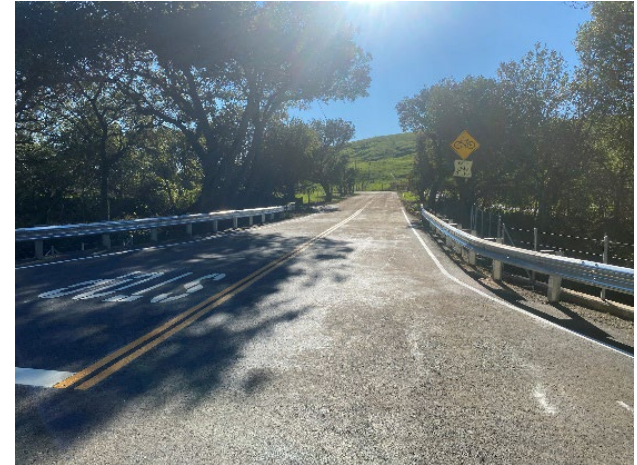
Buhman Ave. Bridge Replacement →
