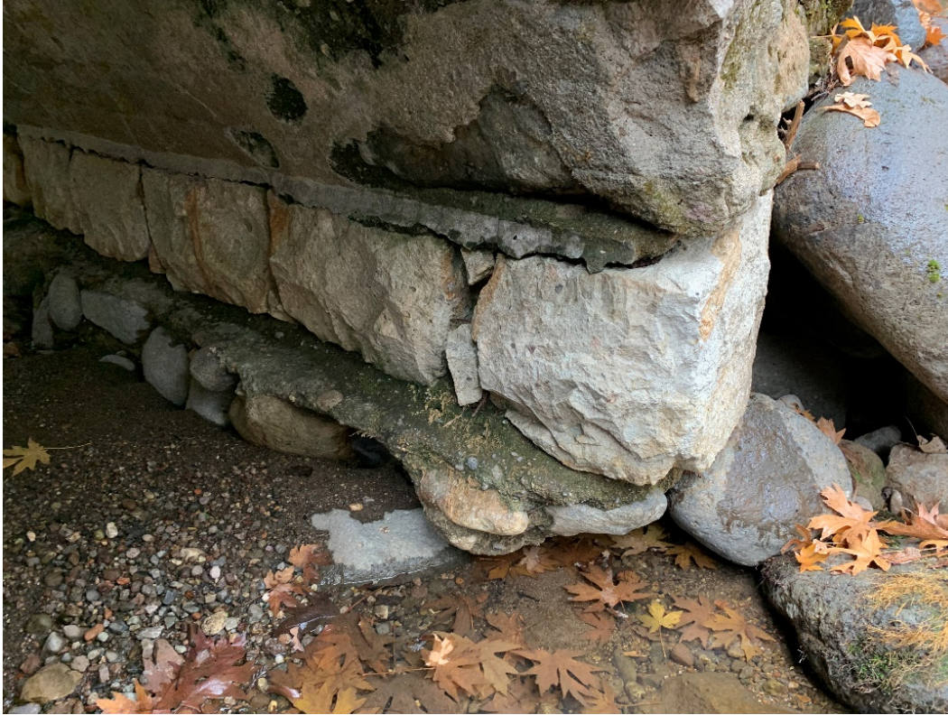
Photo 6: Partially Undermined Foundation at Upstream East Wall
