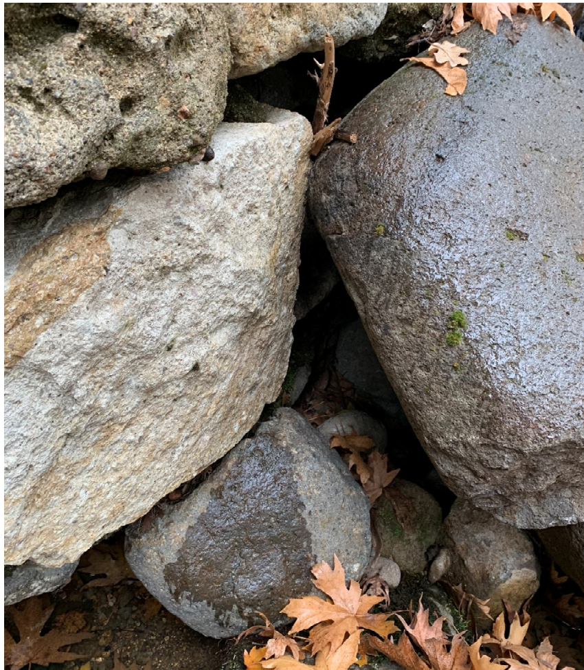
Photo 7: Missing Mortar and Loose Masonry
