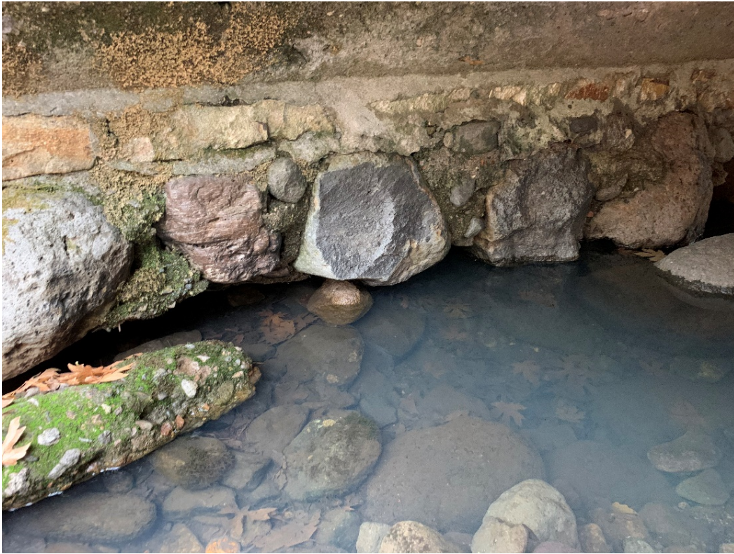
Photo 5: Partially Undermined Foundation at West Wall
