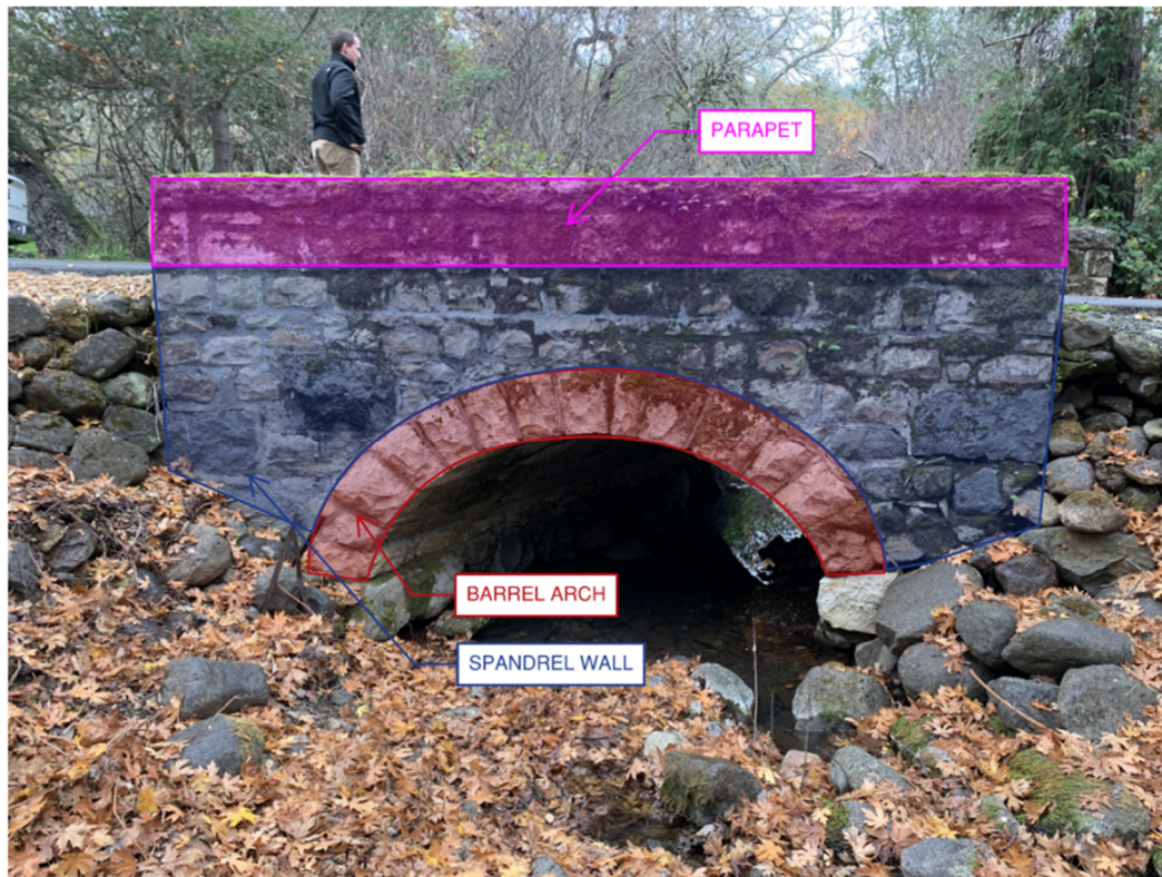
Photo 1: Labeled Elevation View
