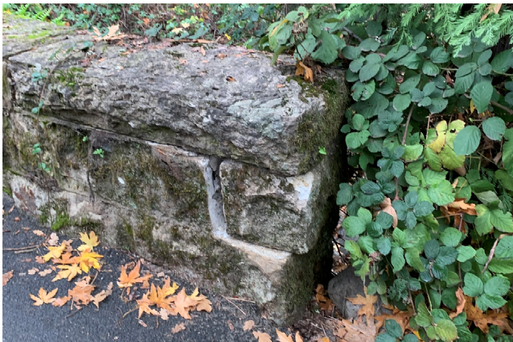
Photo 8: Loose Stone at Parapet
