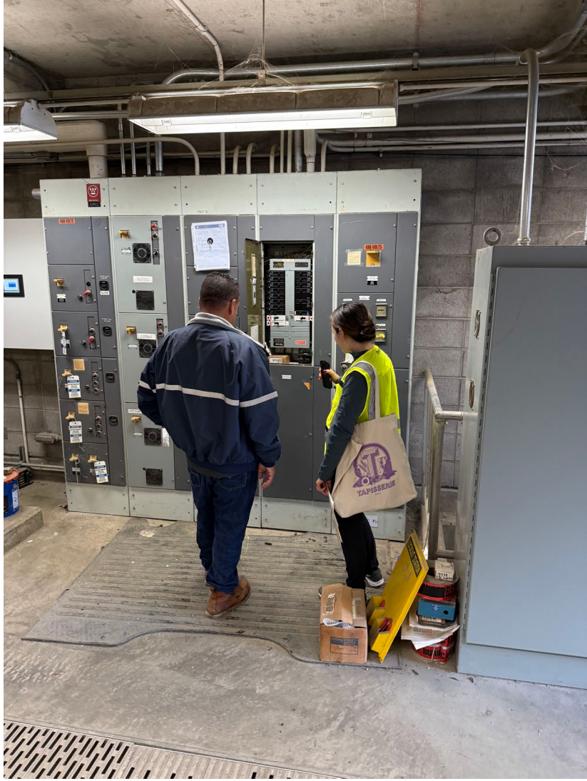
American Canyon Staff & CLEAResult Staff inspecting electrical equipment at future Napa River Ecology Center
