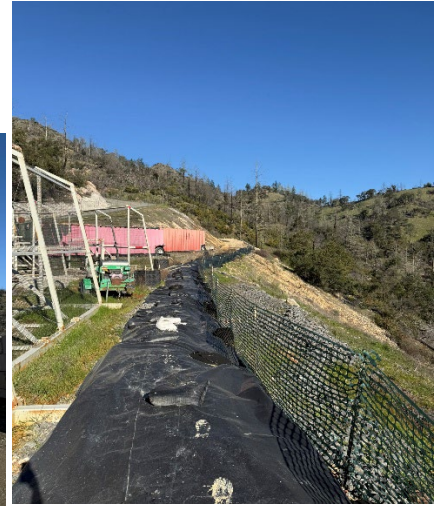
Berm across from Module 5B
