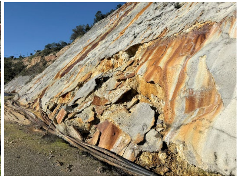
Posi shell damage above Module 5B
