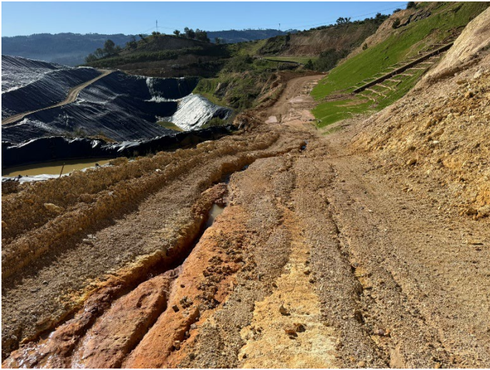
Roadway below landslide, rilling from runoff (looking W)
