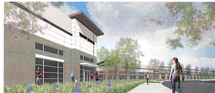
C: VIEW EAST OF BUILDING A MAIN ENTRY AND BUILDING B
