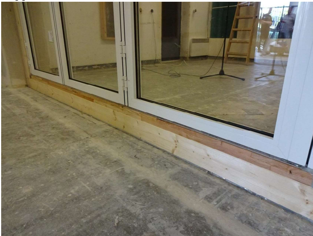
Photo 5: Folding glass wall Acoustic SL70, detail flush sill
