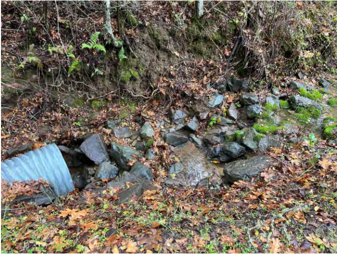
Photo 5: Culvert flow during precipitation.
