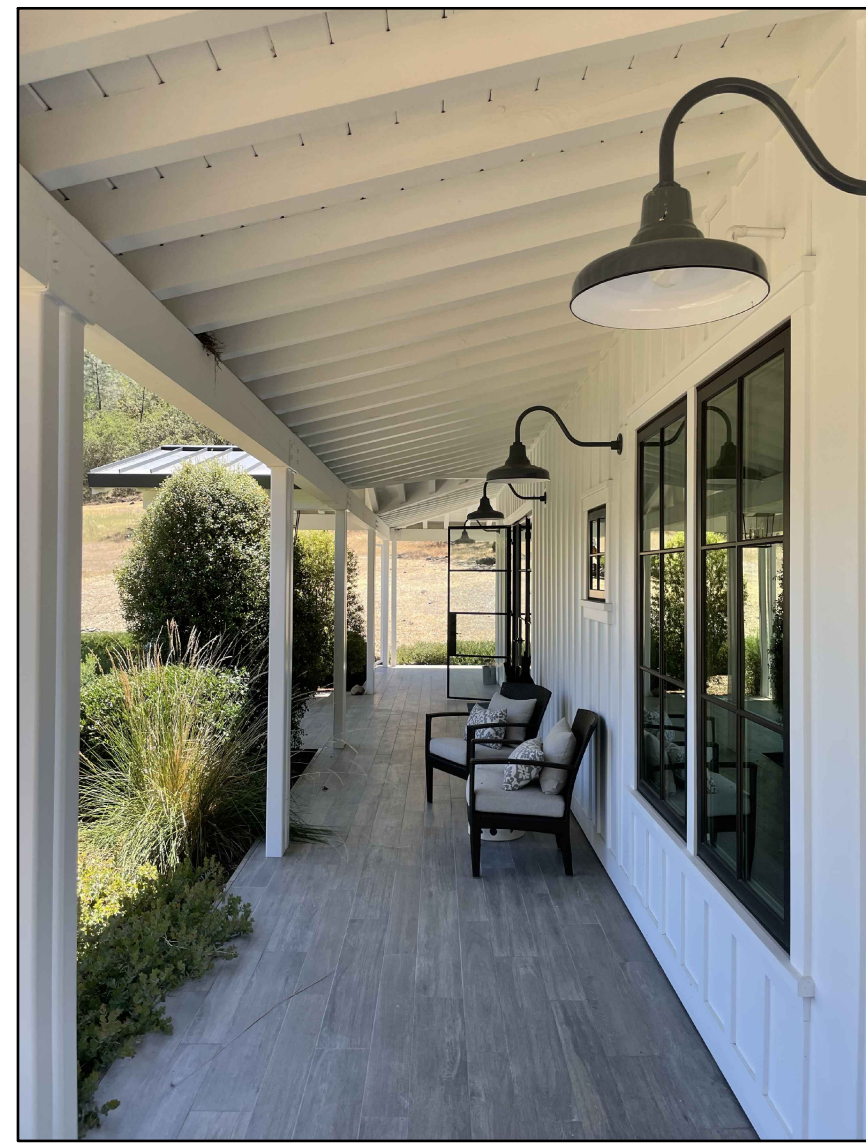
COVERED PORCH LOOKING SOUTH
