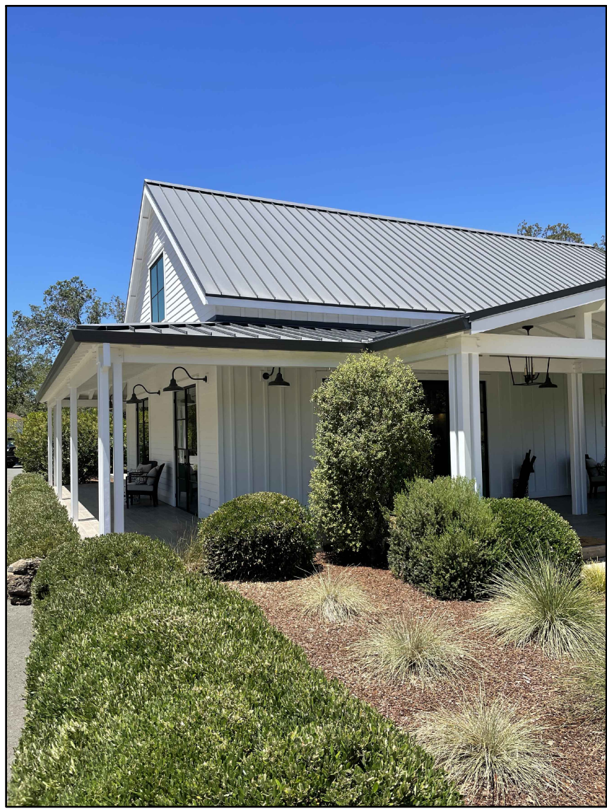
VIEW OF SOUTH FACADE LOOKING EAST
