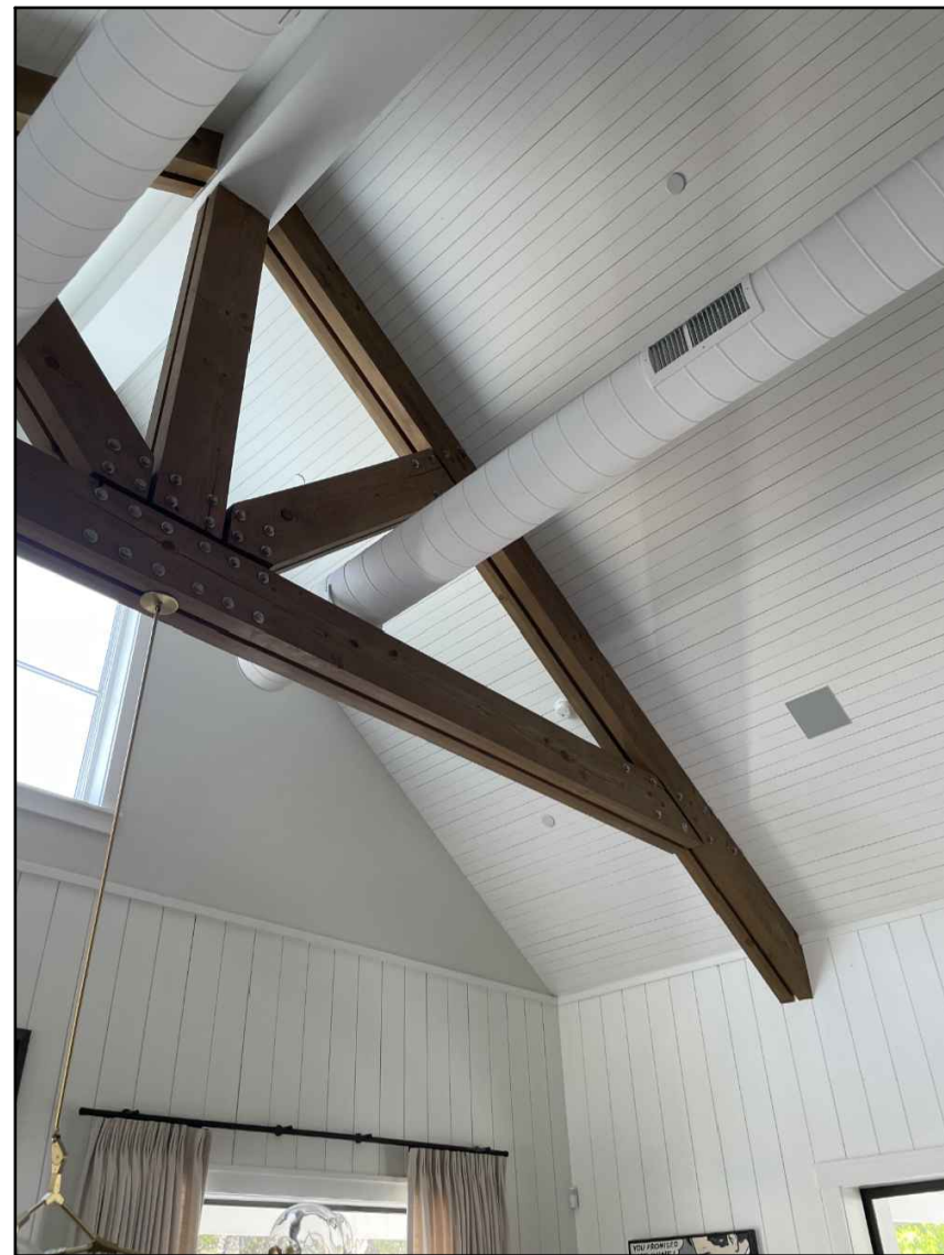
GREAT ROOM EXPOSED TRUSSES & CEILING TREATMENT
