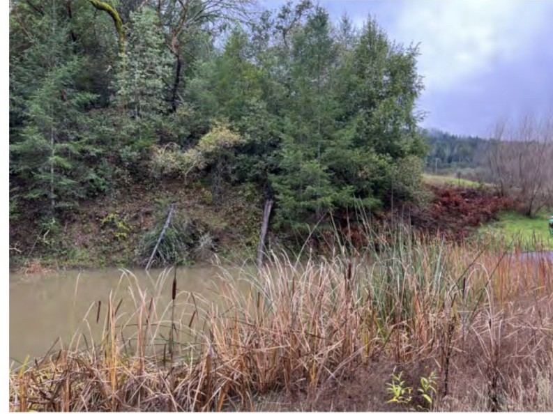
Photo 4: Detention Basin (Lower)
