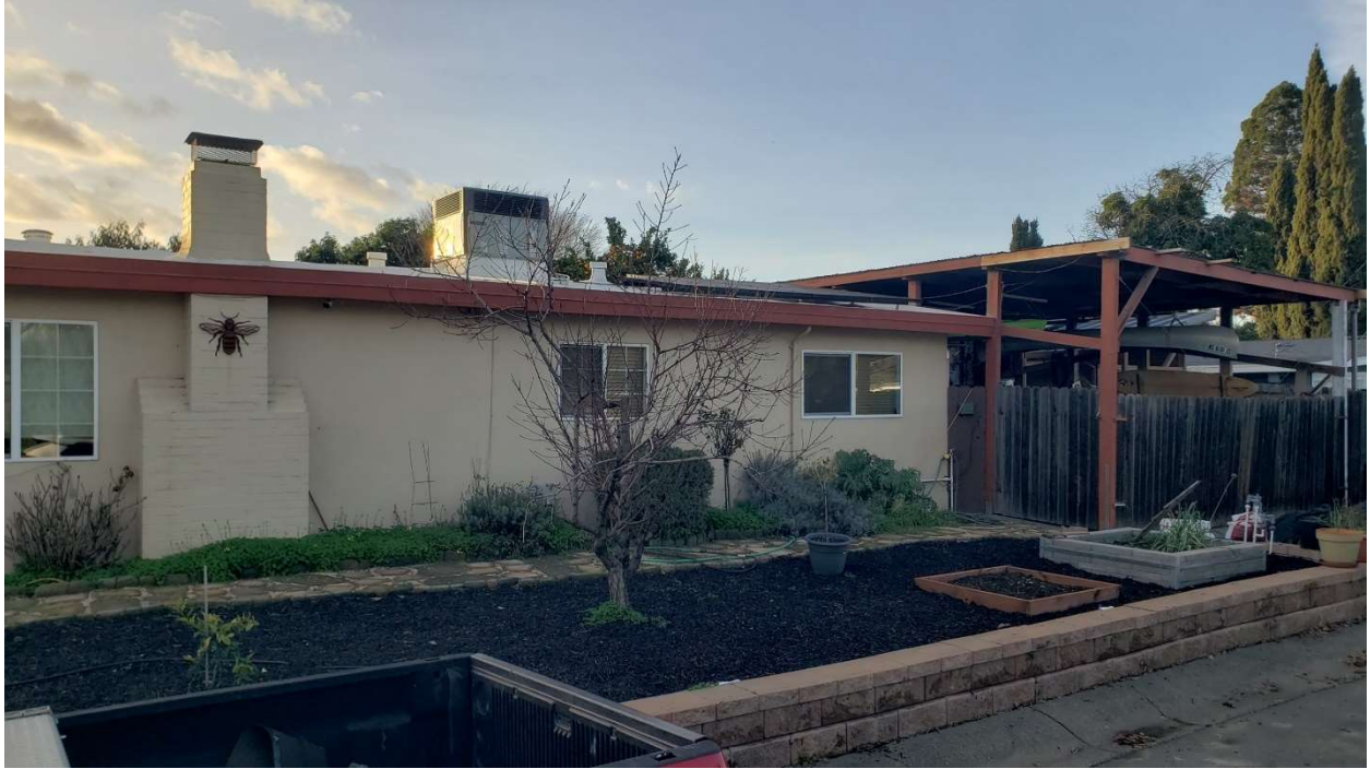
Figure 4: Carport seen to the right of house. Structure to be demolished.
