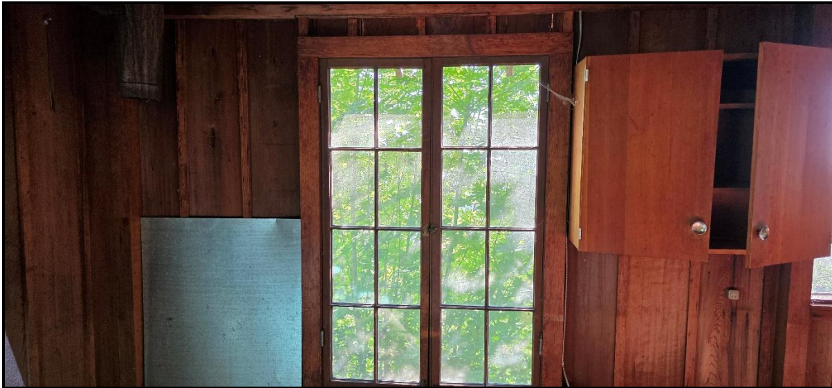
Figure 6. View of the two-by-four light window in the small cabin.
