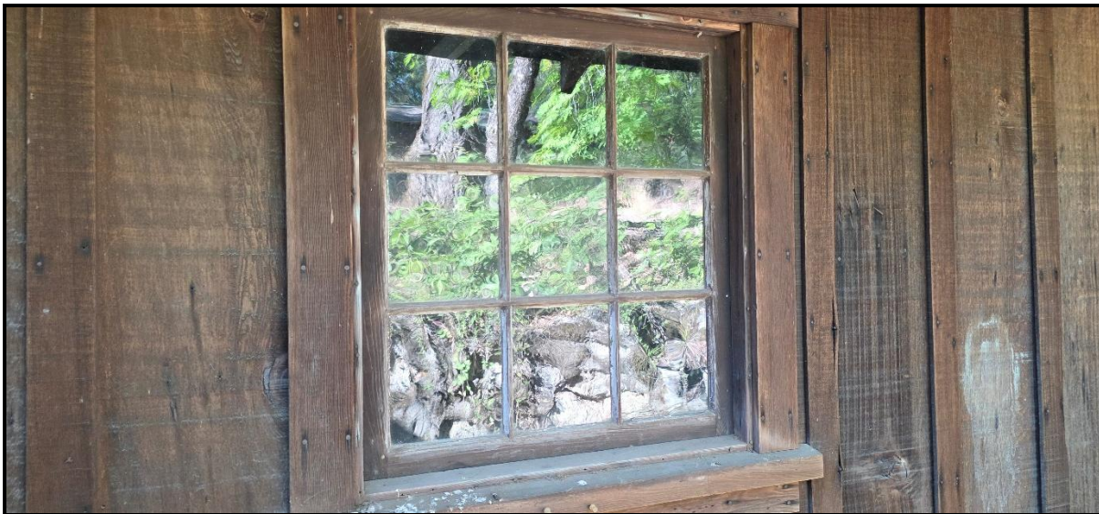
Figure 5. Example view of the three-by-three light windows in the small cabin.
