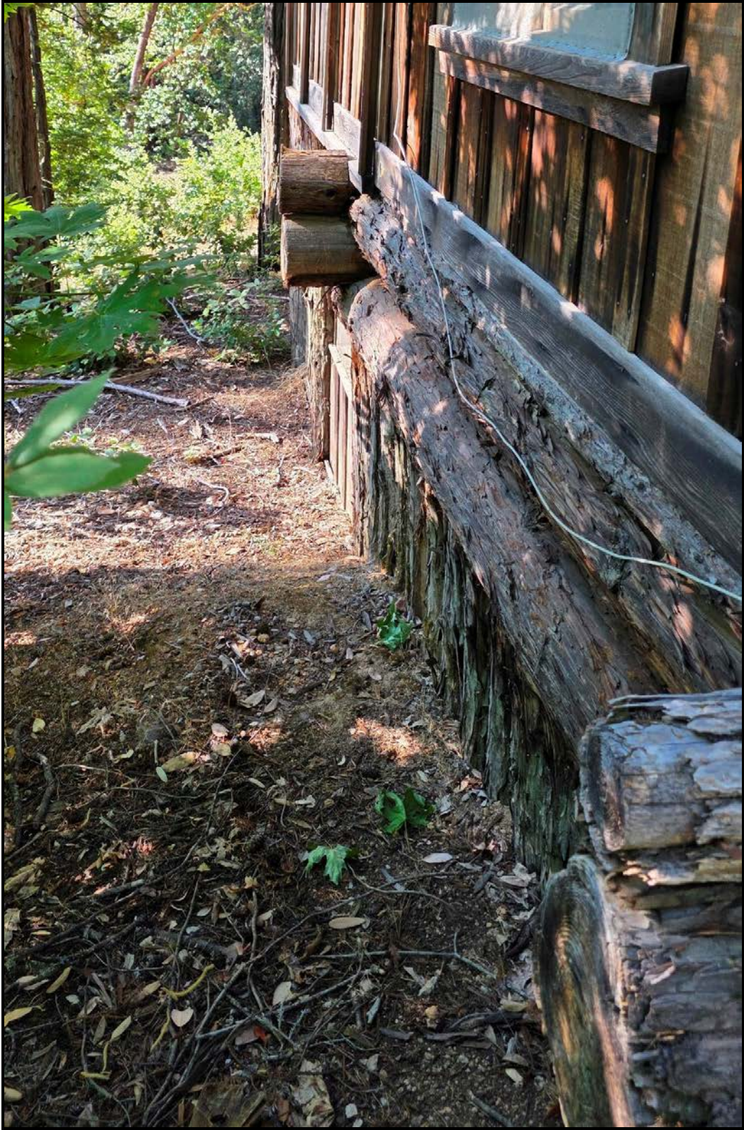
Figure 3. View of the east elevation of the small cabin showing the unhewn interlocking log foundation.
