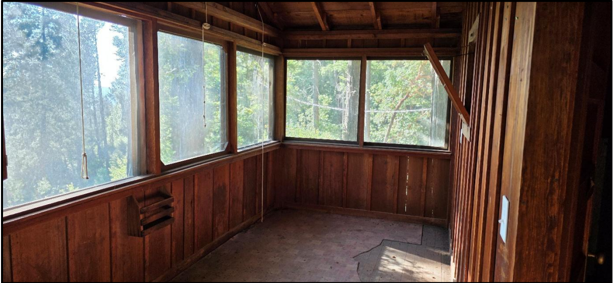
Figure 7. View of the ribbon of single-paned windows in the small cabin.
