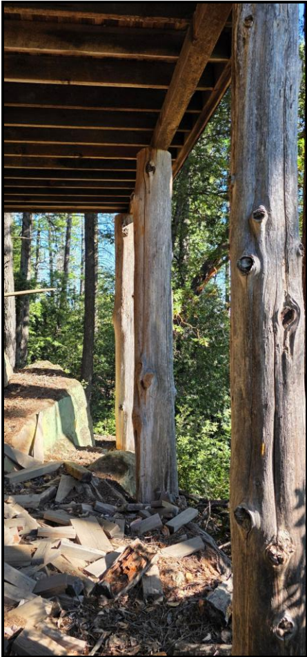
Figure 9. View of the pole foundation posts.
