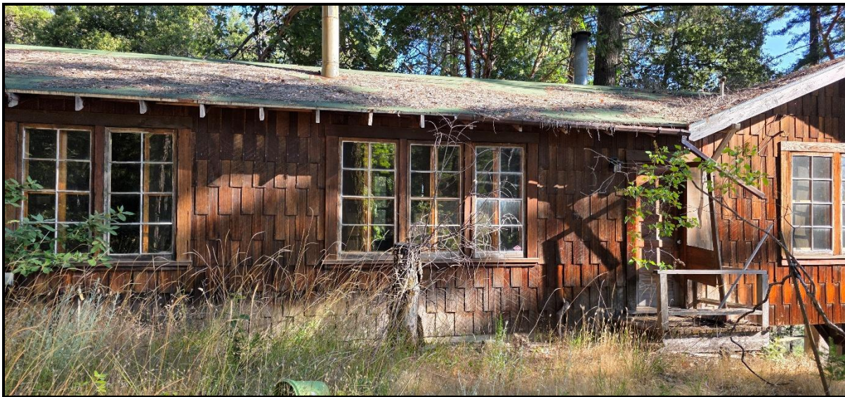
Figure 11. Example view of the windows on the large cabin.
