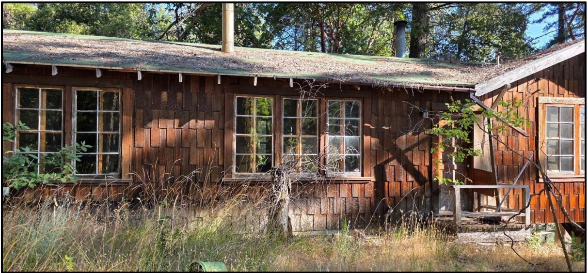
Figure 14. Example view of the windows on the large cabin.
