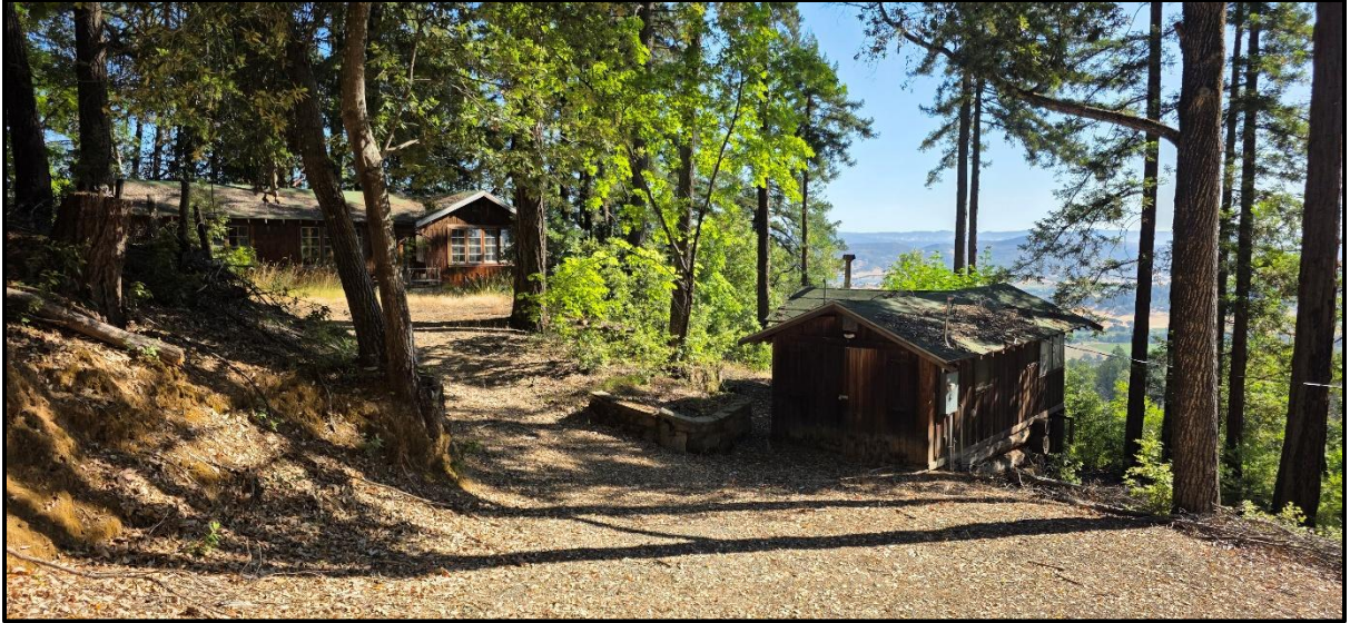
Figure 3. View of the Bade Cabins, facing northeast.
