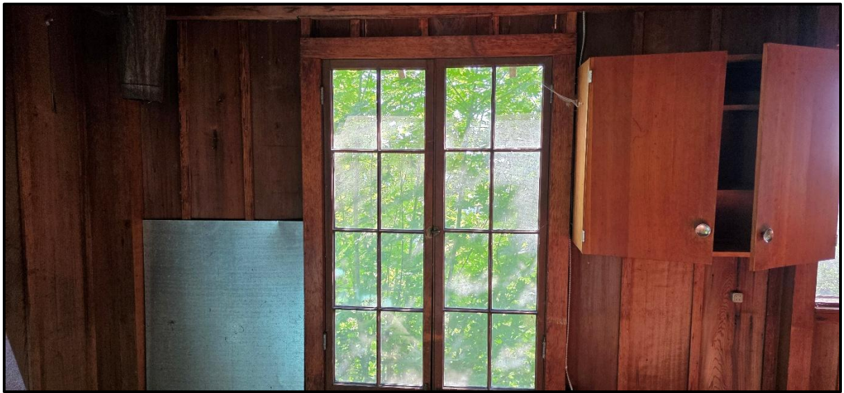
Figure 9. View of the two-by-four light window in the small cabin.
