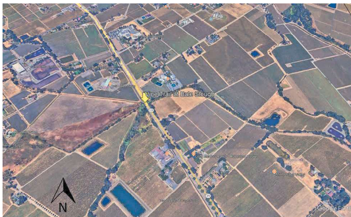
Figure 1. Aerial view of project location at Bale Slough crossing under State Highway 29, Napa County, California. Bale Slough flows west to east, draining from Bear Canyon toward the Napa River. (Source: Google Earth, 2025)
