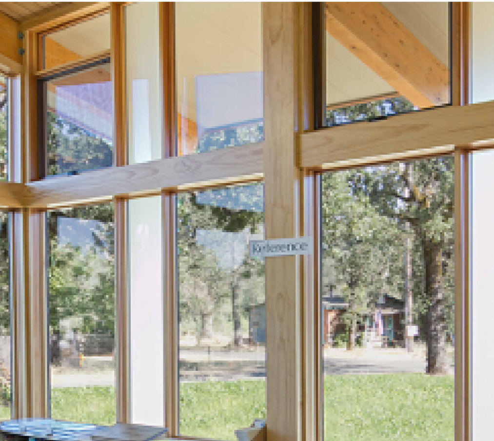
ALUMINUM CLAD WOOD WINDOW WALL
