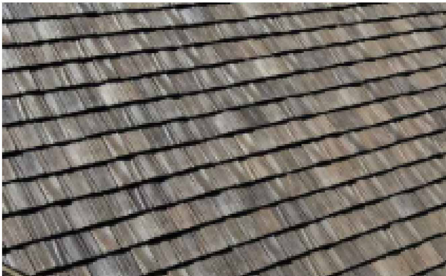
COMPOSITION SHINGLE ROOFING
