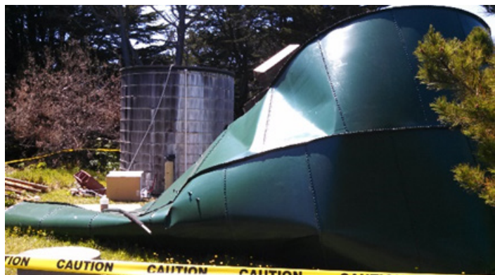
Figure 3: Failed epoxy coated bolted steel water tank (Pacific Reefs Water District)
