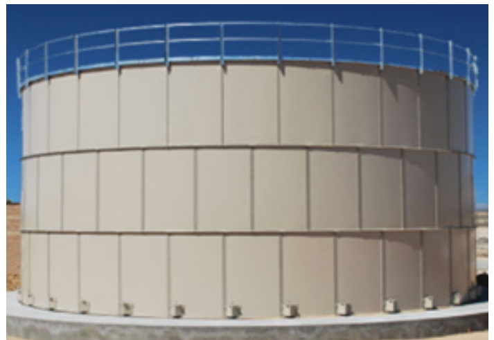
Figure 2: Typical Bolted Carbon Steel Tank
