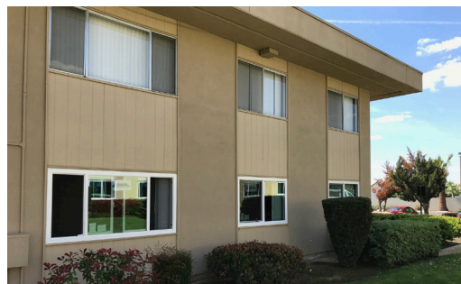
Comparison of old windows vs. new dual-pane windows at North Park Apartments in Oildale, CA.
