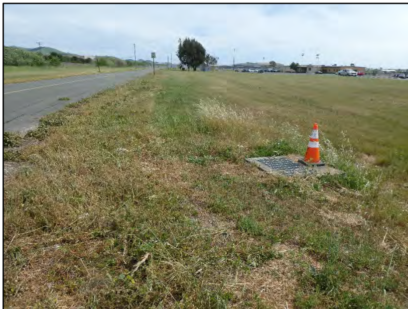
Site photo – Photo point #8
