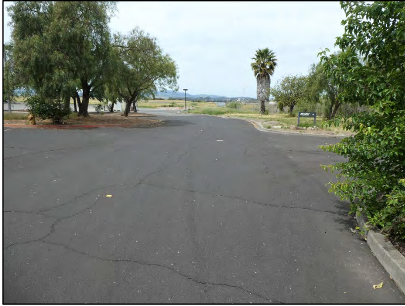
Site photo – Photo point #3
