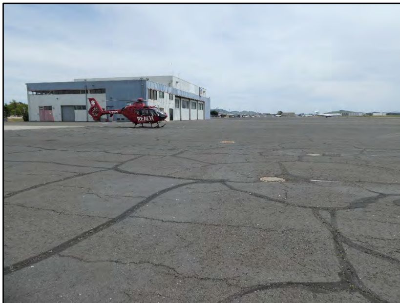
Site photo – Photo point #4
