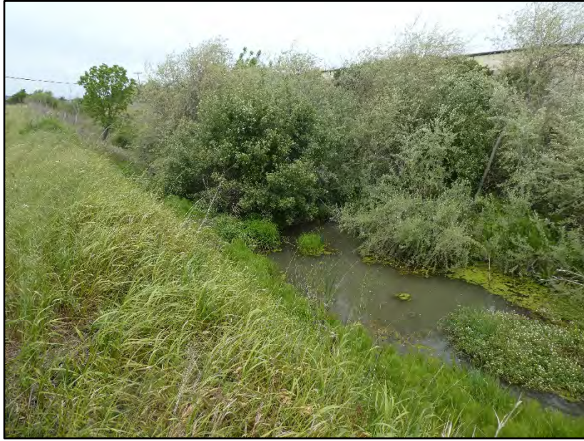
Site photo – Photo point #1
