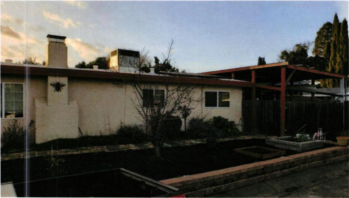
Figure 4: Carport seen to the right of house. Structure to be demolished.
