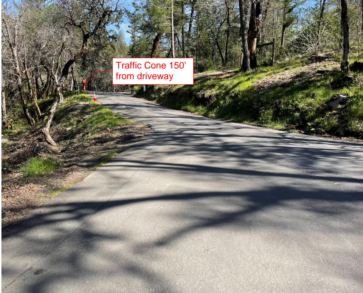
Photo taken 15 ft back from edge of roadway in existing driveway looking Northeast
