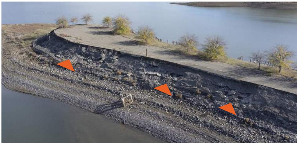
**C** STRUCTURAL DAMAGE ON CONCRETE RETAINING WALL OF PENINSULA
