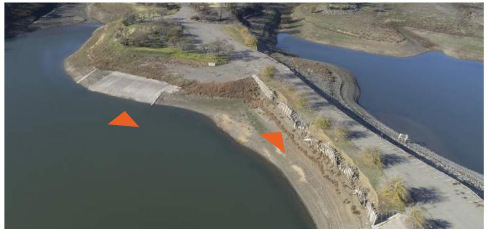
**D** EXISTING BOAT RAMP & WOOD RETAINING WALL IN DISREPAIR
