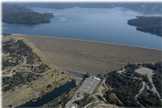
Lake Oroville Dam
