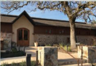
EXISTING STONE WINERY BUILDING
