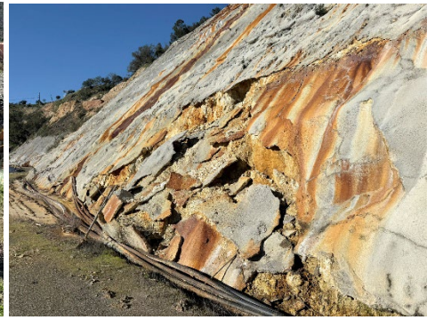
Posi shell damage above Module 5B
