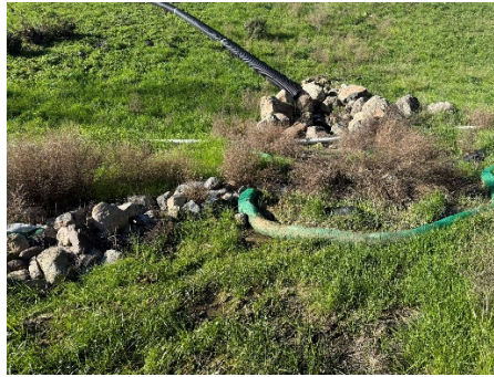
Stormwater conveyance outlet
