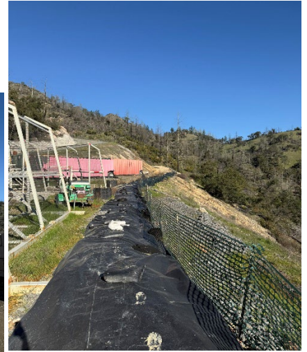
Berm across from Module 5B
