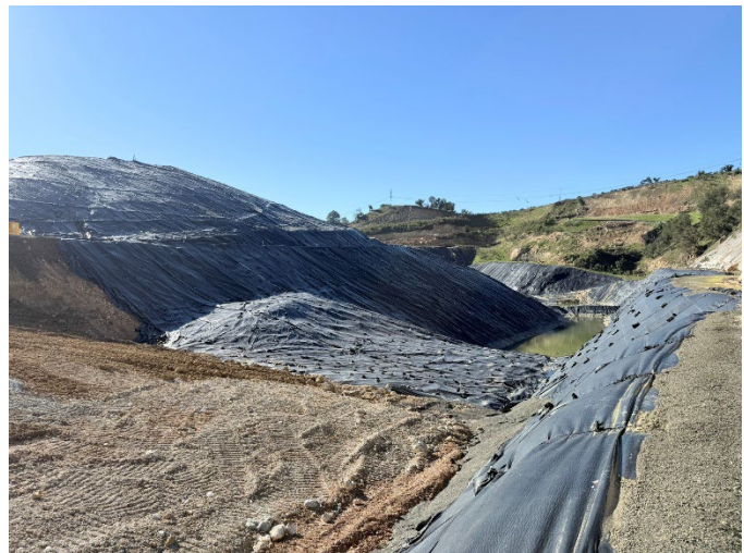
Module 5B- end of filled area with cover, and stormwater pond
