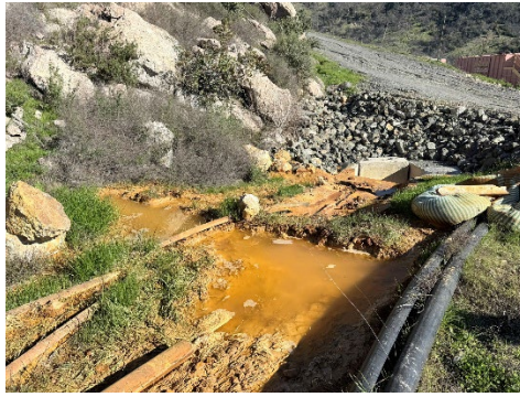
Stormwater holding prior to discharge
