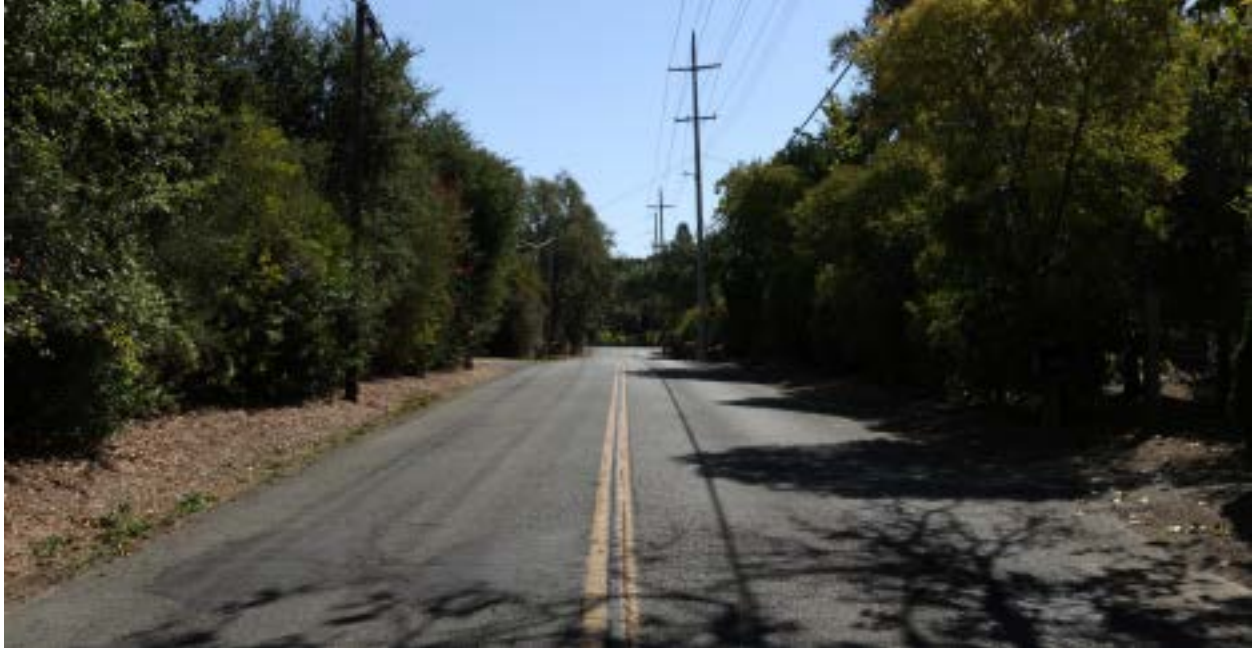
3E. No Pedestrian or Bike Facilities on Hedgeside Ave, Approaching Monticello Road
