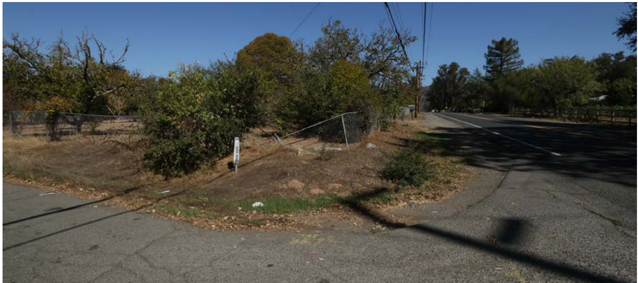
5C. Photo of Damage from Unprotected Left Turn on Monticello
