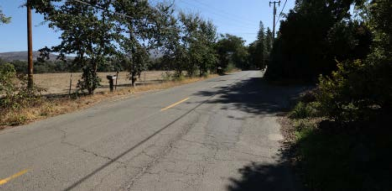
3C. No Pedestrian or Bike Facilities on Hedgeside Ave
