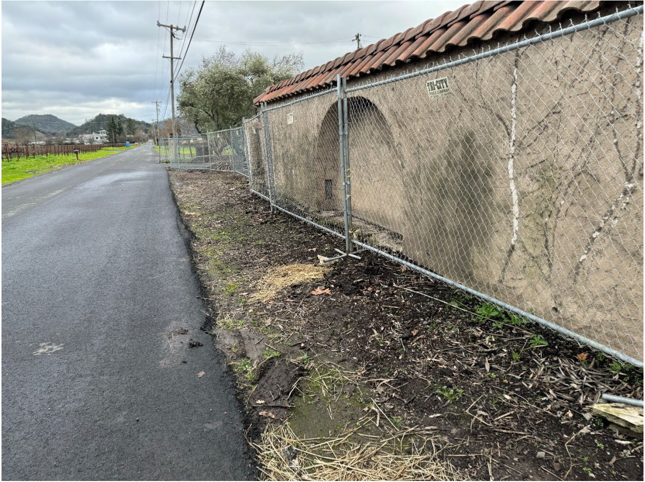
View of Existing Privacy Wall Adjacent to State Lane
