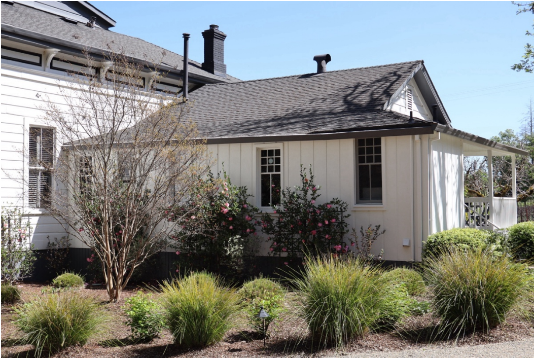
Figure 24. North elevation of the 1883 house, with the 1932 hipped addition, facing south.
