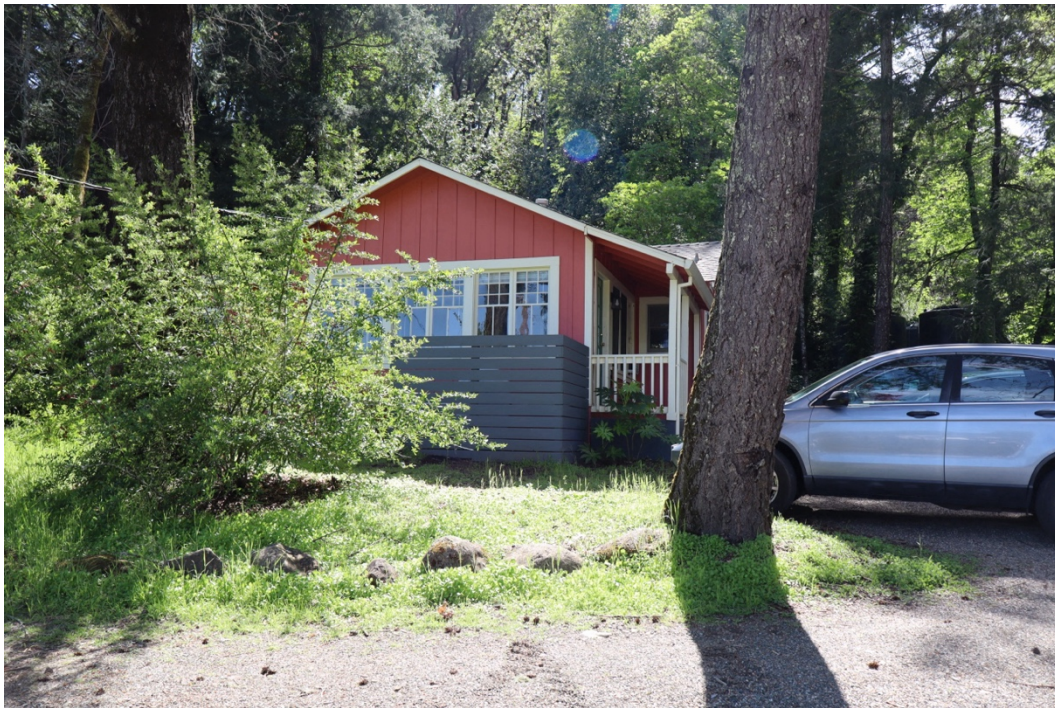
Figure 31. East elevation, facing west.
