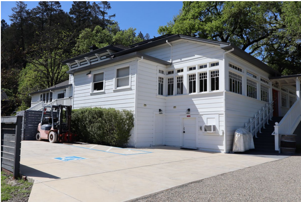
Figure 4. South elevation, facing northwest.
