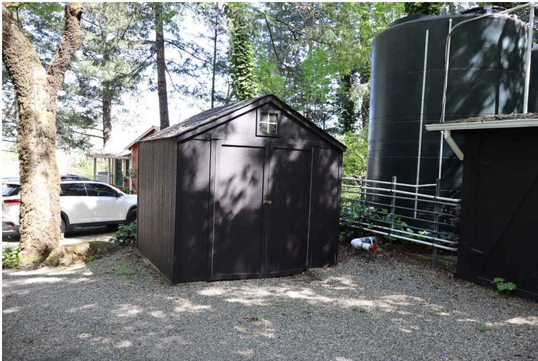
Figure 50. Front-facing gable shed, next to five water tanks.
