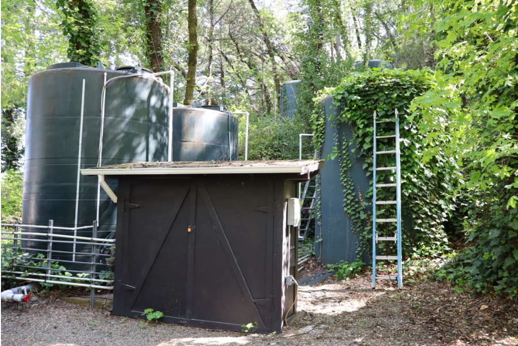
Figure 49. Five above-ground water tanks and a shed.
