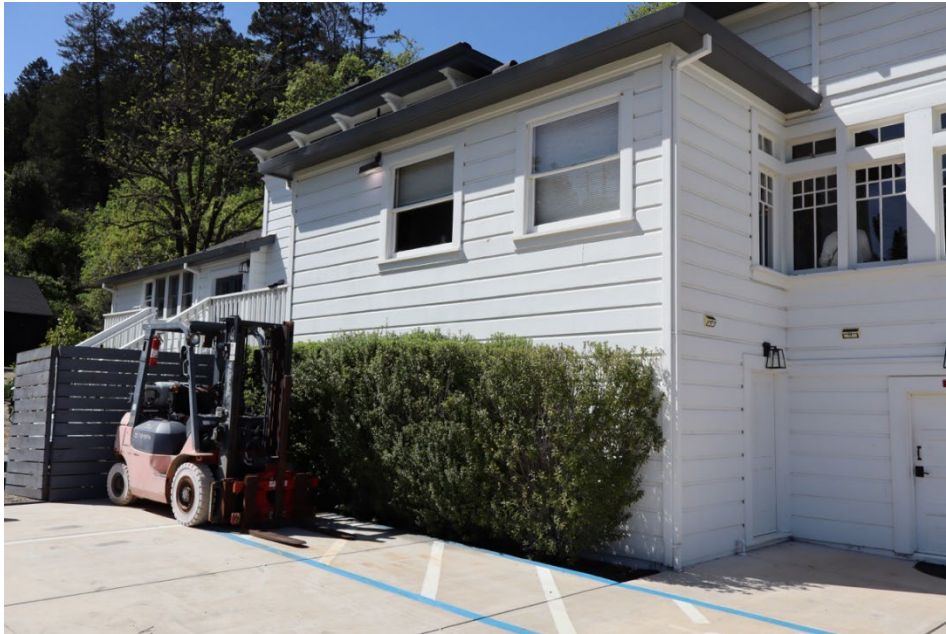
Figure 5. South elevation, facing northwest.
