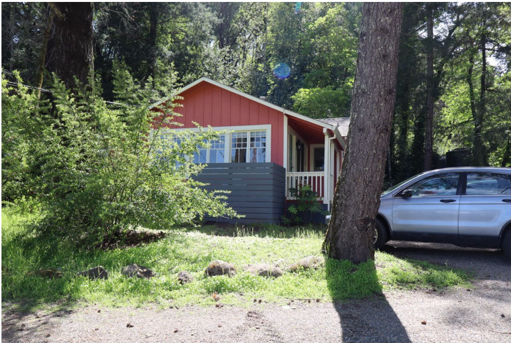
Figure 18. East elevation, facing west.
