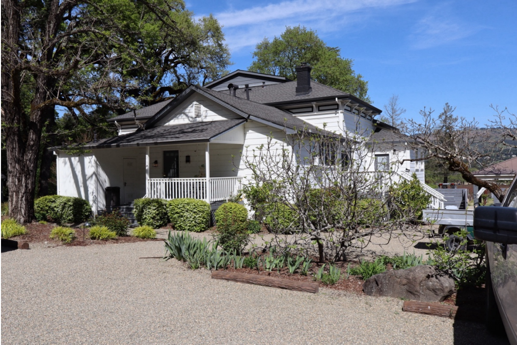
Figure 21. West and south elevations of the 1883 house, with ca. 1905, 1932, and 1950s additions, facing northeast.
