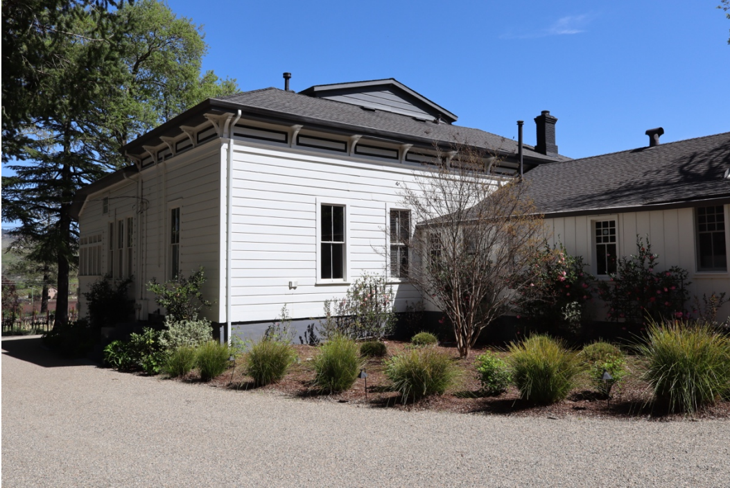
Figure 23. West and north elevations of the 1883 house, with ca. 1905 and 1932 additions, facing southeast.
