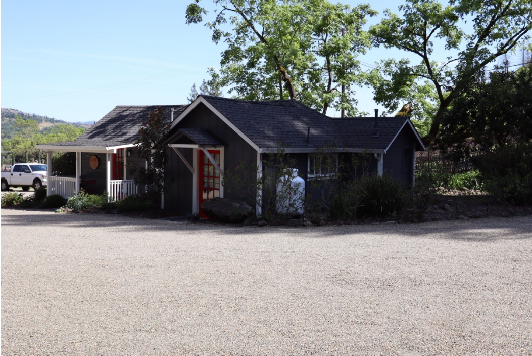
Figure 35. North and west elevations, facing southeast.
