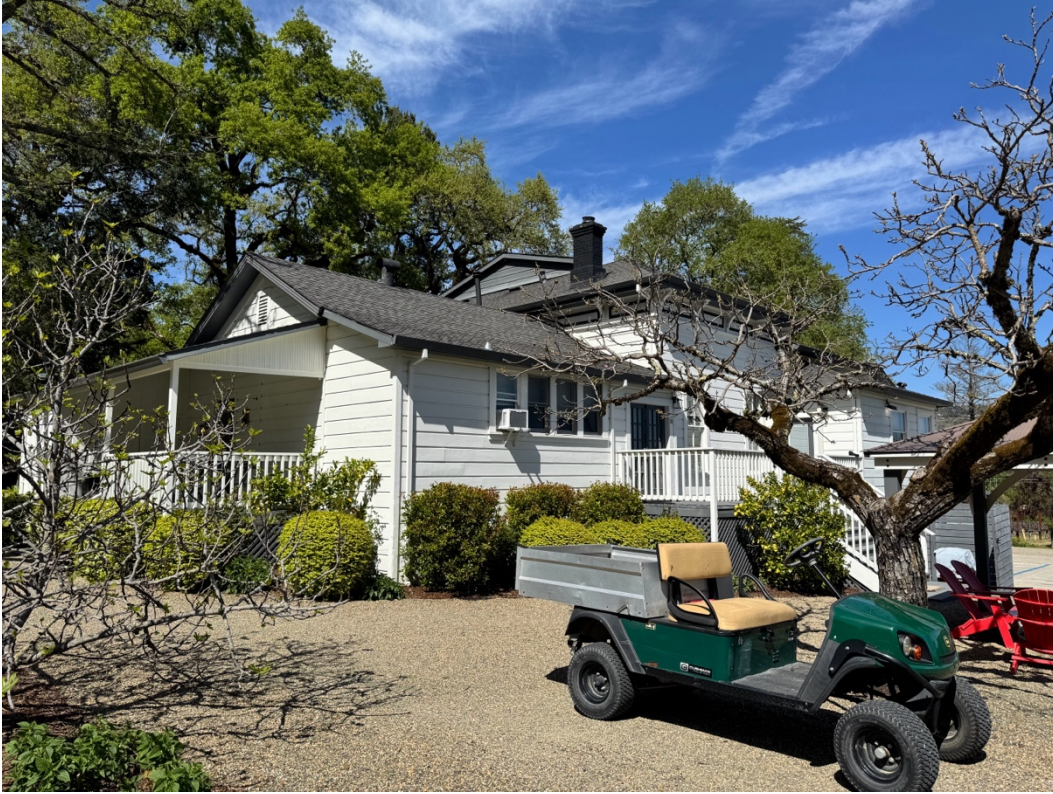
Figure 19. South and west elevations, facing northeast.
