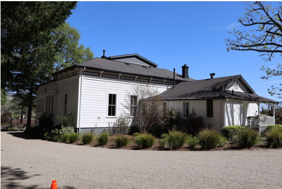
Figure 9. West and north elevations of 1883 house, with ca. 1905 and 1932 additions, facing southeast.
