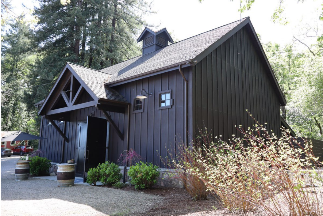
Figure 27. East elevation and north elevations, facing southwest.
