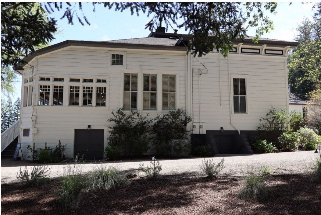
Figure 12. North elevation, with ca. 1905 and 1932 additions, facing southwest.
