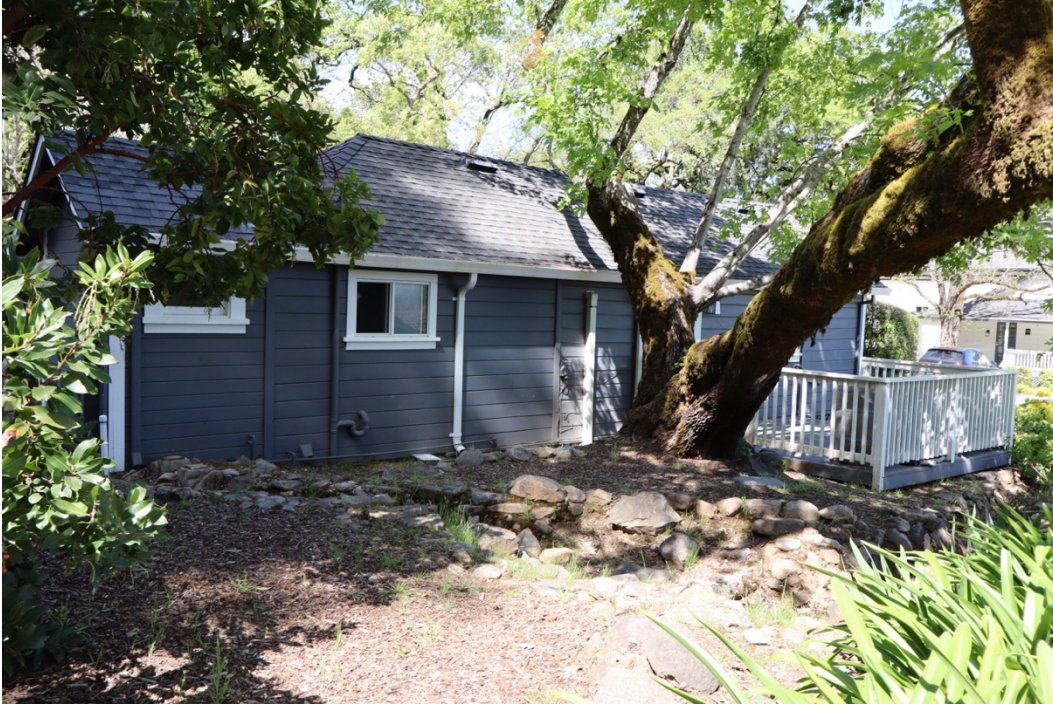
Figure 37. South elevation, facing north.
