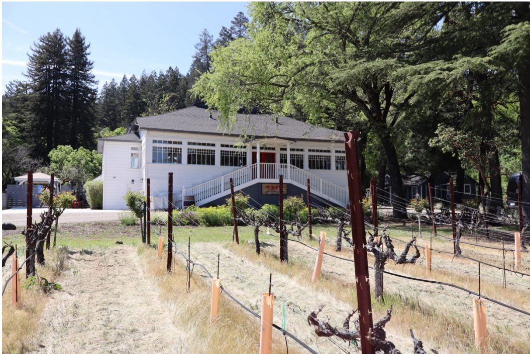
Figure 15. East elevation, facing west.
