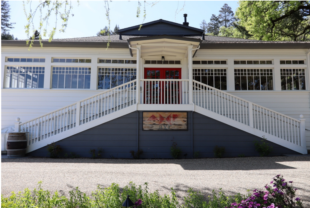
Figure 16. East elevation, facing west.
