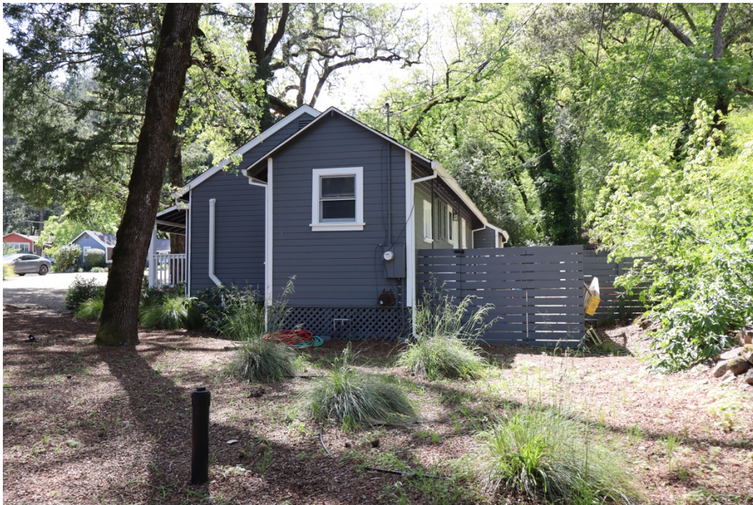
Figure 28. East and north elevations, facing southwest.
