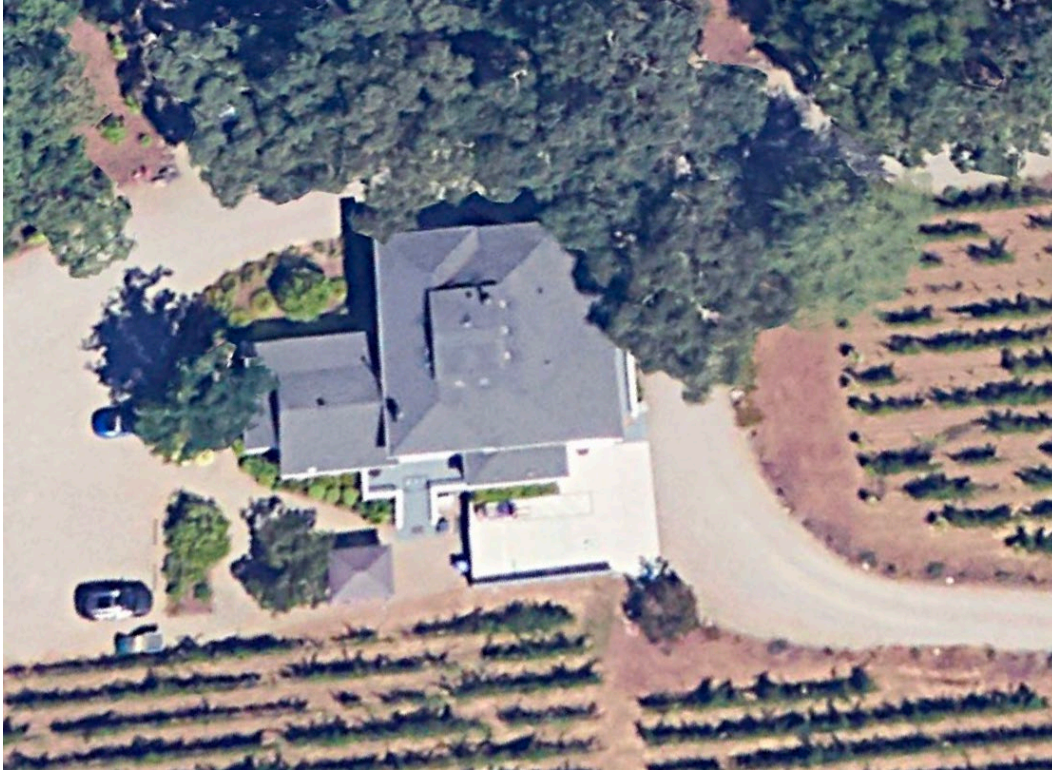
Figure 1. 1883 house with four phases on construction, with the 1883 section in yellow, ca. 1905 addition in red, 1932 additions in blue and 1950s additions in green.
