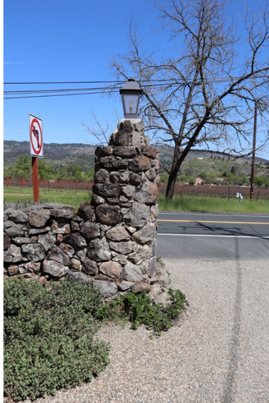
Figure 43. Detail of stone pillar at entrance with lantern, facing east.
