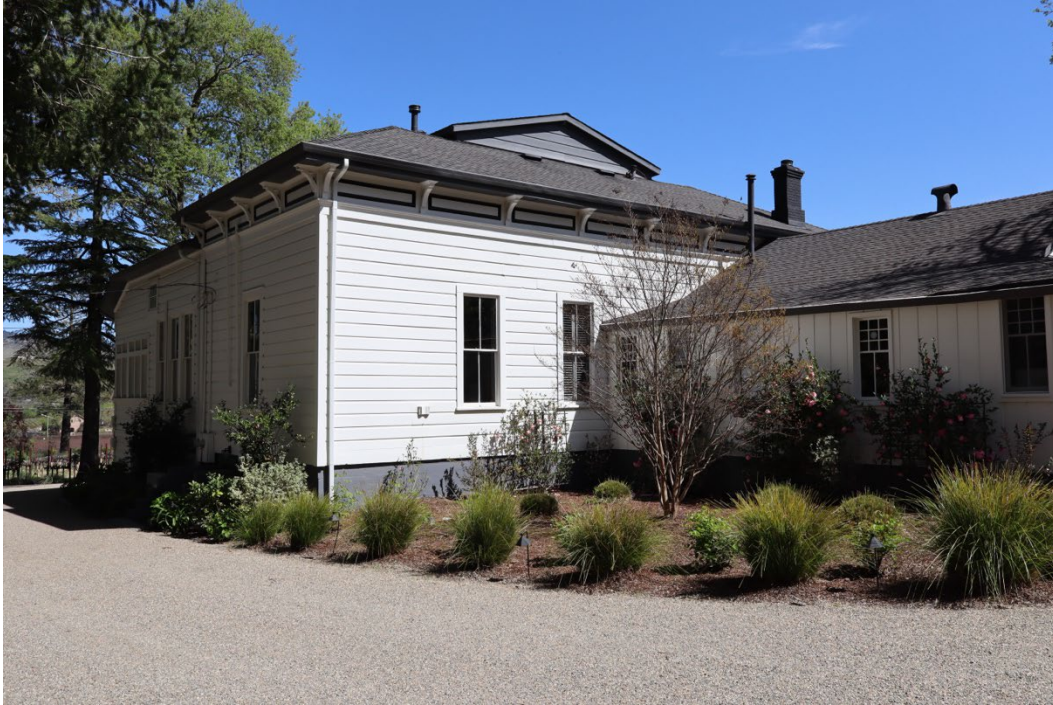
Figure 10. West and north elevations of the 1883 house, with ca. 1905 and 1932 additions, facing southeast.
