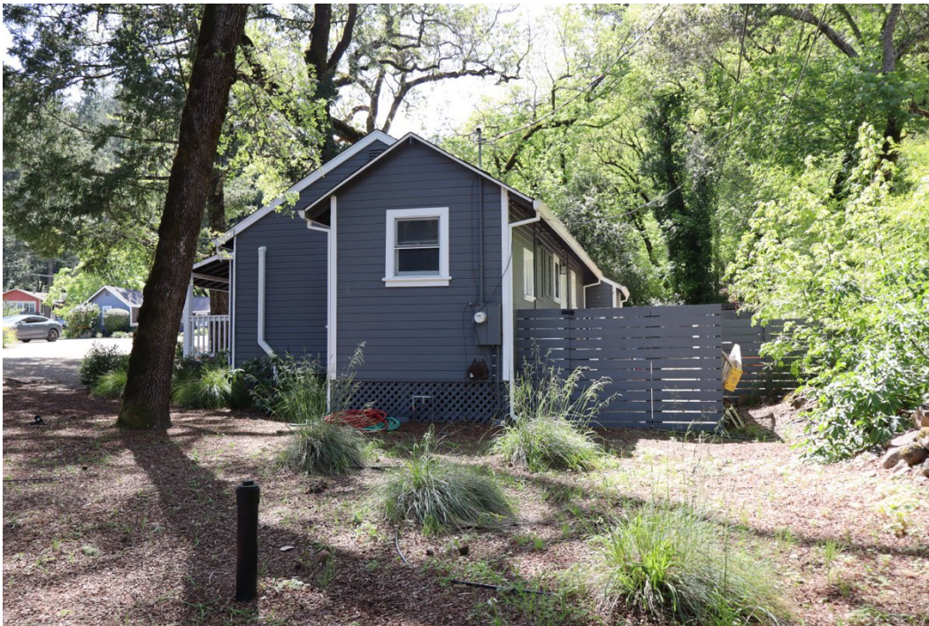
Figure 15. East and north elevations, facing southwest.
