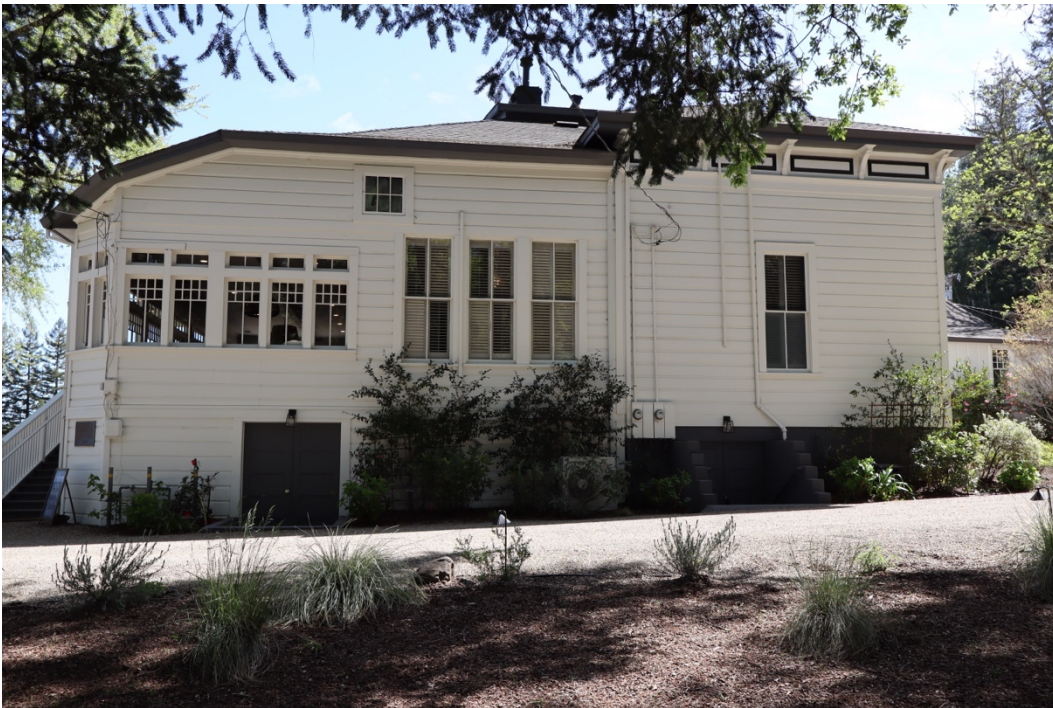
Figure 25. North elevation, with ca. 1905 and 1932 additions, facing southwest.
