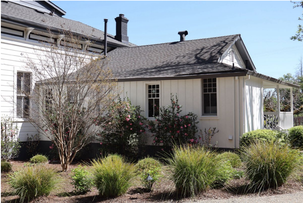
Figure 11. North elevation of the 1883 house, with the 1932 hipped addition, facing south.
