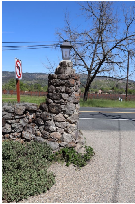
Figure 30. Detail of stone pillar at entrance with lantern, facing east.
