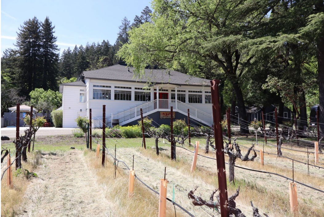
Figure 2. East elevation, facing west.
