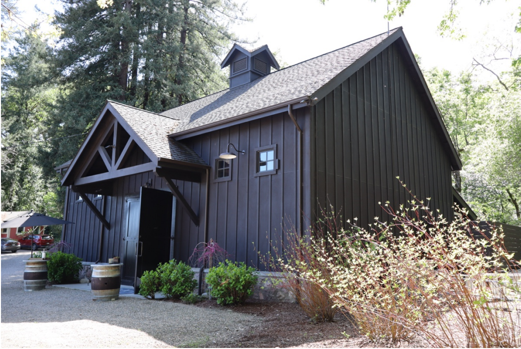
Figure 40. East elevation and north elevations, facing southwest.
