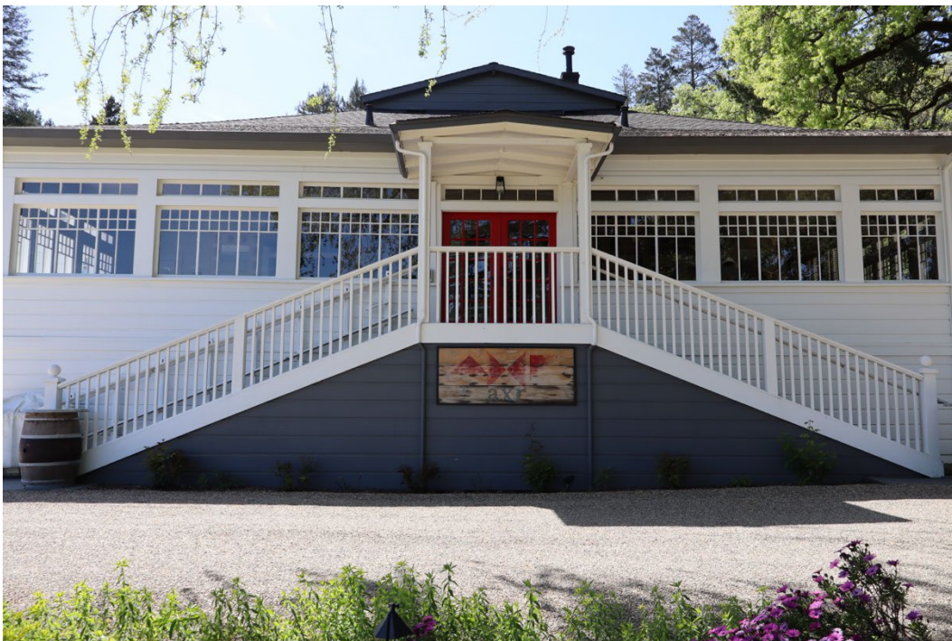
Figure 3. East elevation, facing west.
