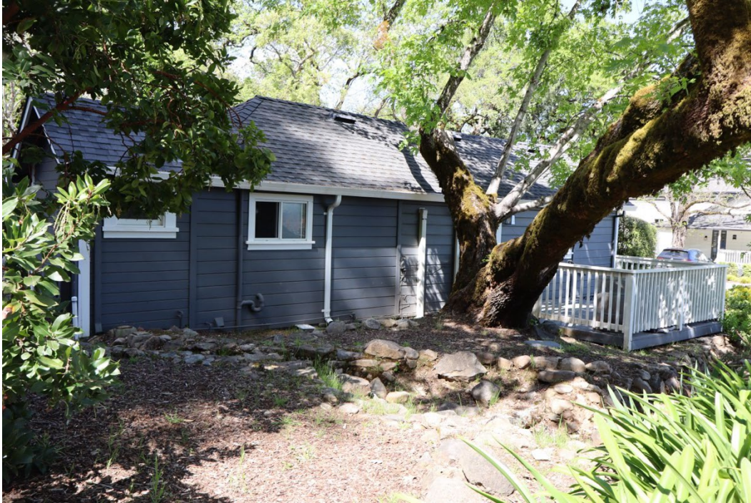
Figure 24. South elevation, facing north.
