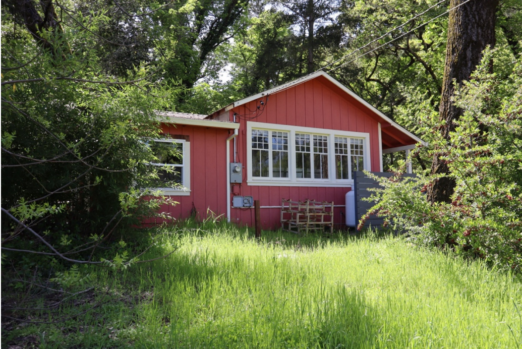
Figure 32. East elevation, facing west.
