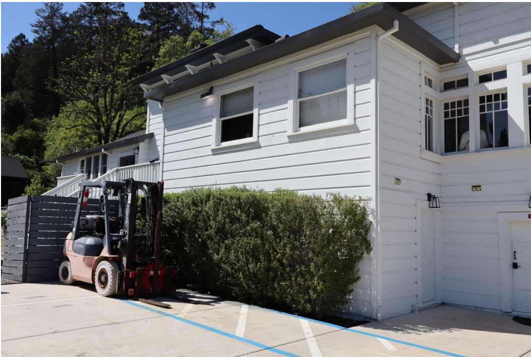
Figure 18. South elevation, facing northwest.
