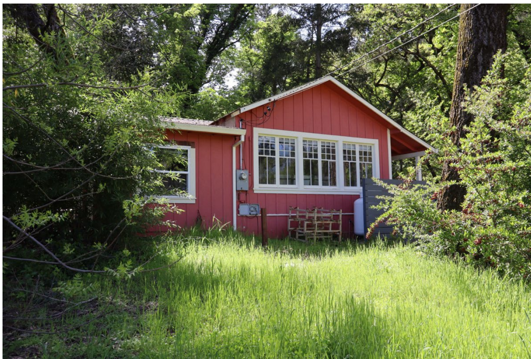
Figure 19. East elevation, facing west.
