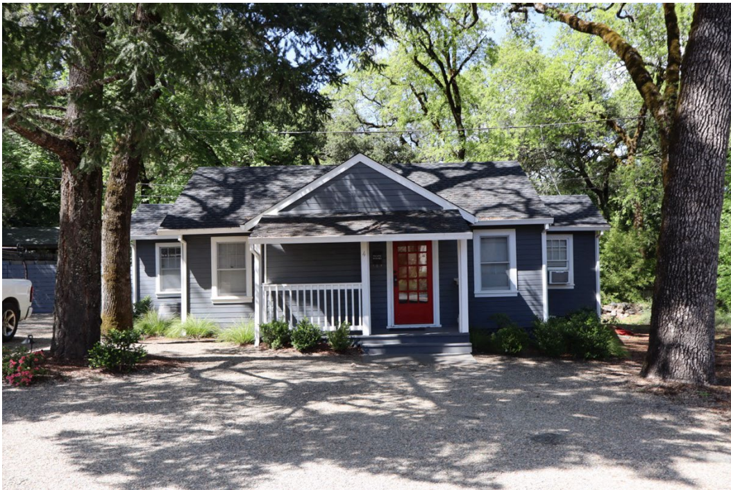
Figure 13. South elevation, facing north.
