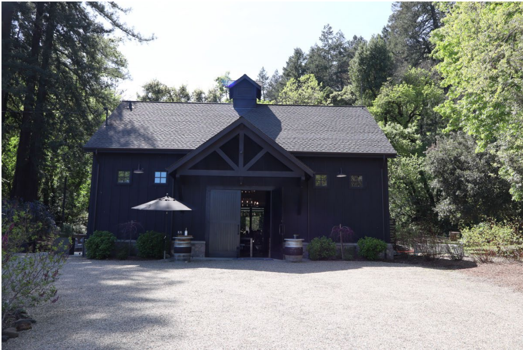
Figure 26. East elevation of ca. 1988 barn, facing west.
