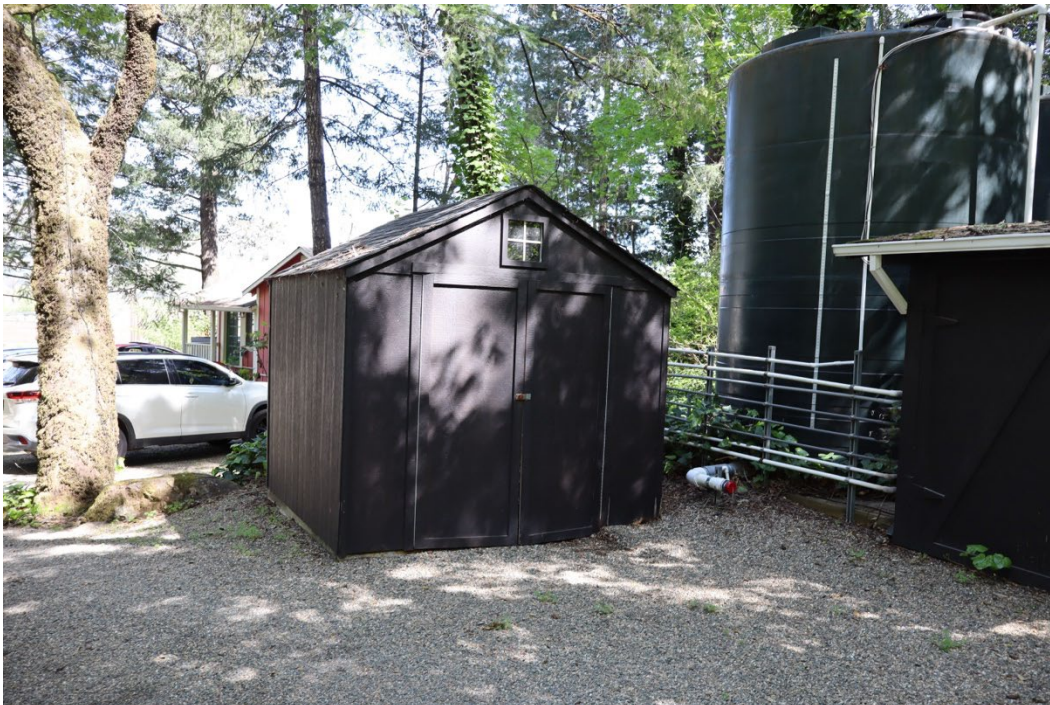
Figure 37. Front-facing gable shed, next to five water tanks.
