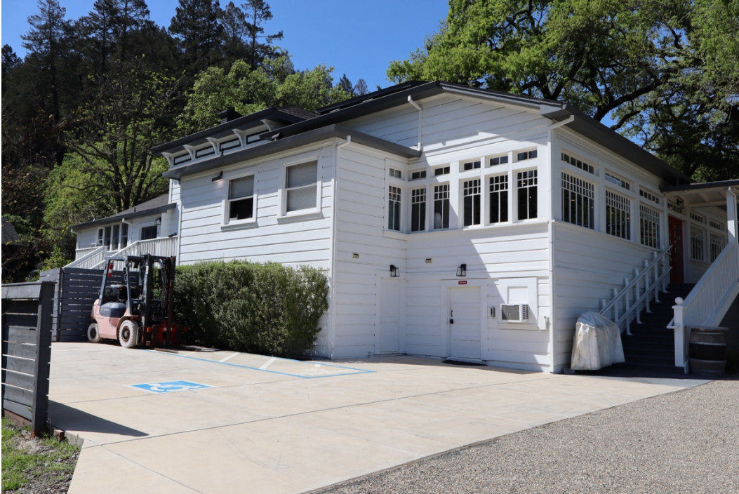
Figure 17. South elevation, facing northwest.
