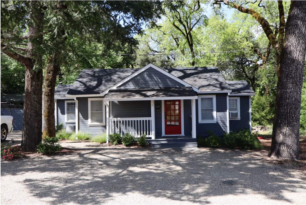
Figure 26. South elevation, facing north.
