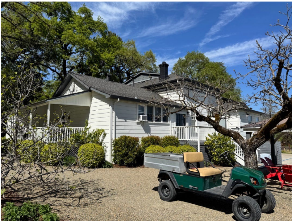
Figure 6. South and west elevations, facing northeast.
