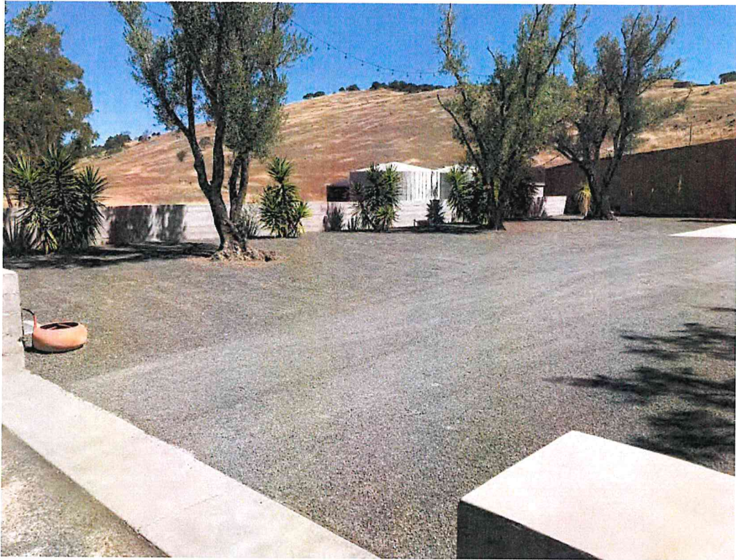
Photo #9 – North Courtyard Parking Area
