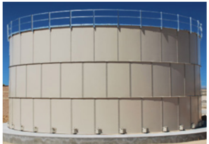
Figure 2: Typical Bolted Carbon Steel Tank
