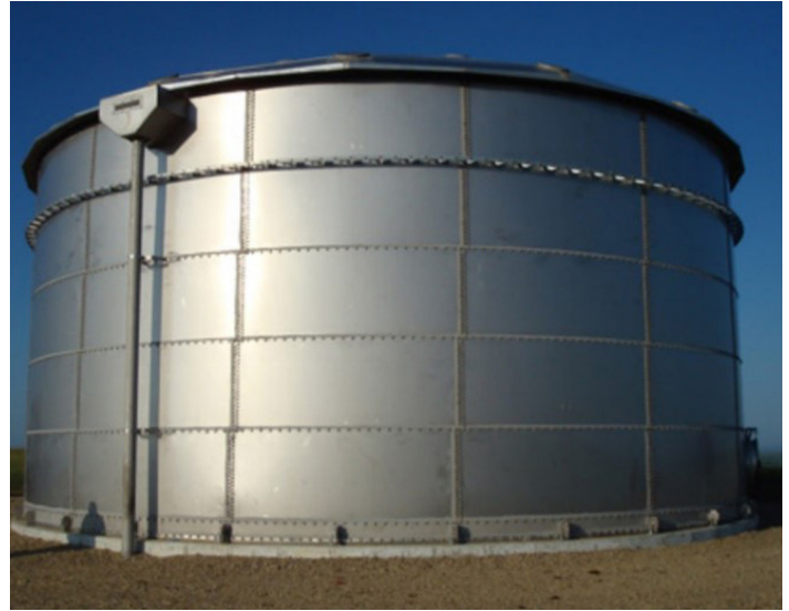
Figure 1: Typical Bolted Steel Tank
