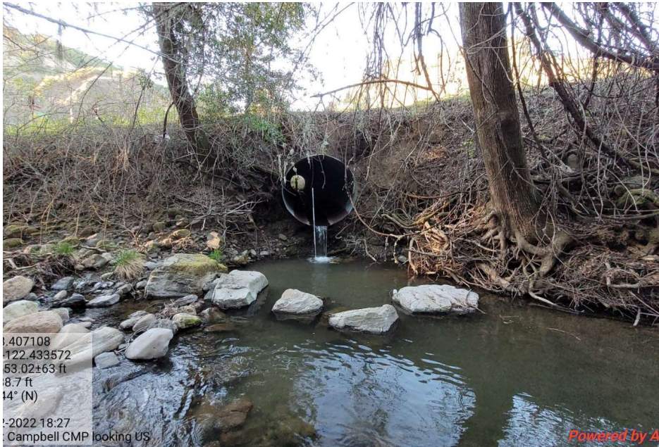
Photo 1. Outlet of the Dry Creek Road Culvert conveying flows from Campbell Creek to Dry Creek.
