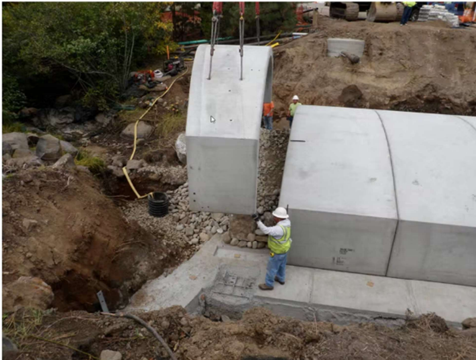
Photo 3 Installation of a Bottomless Arch Bridge Precast Culvert along Third Creek in Incline Village, Nevada
