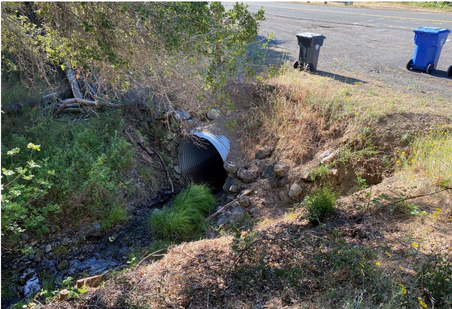
Photo 2. Inlet of the Dry Creek Road Culvert conveying flows from Campbell Creek to under Dry Creek Road.
